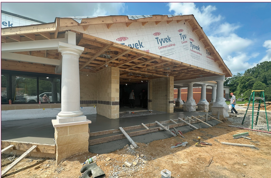
July 16, 2025, concrete poured for entrance and ramp. Both will be covered for easier access to the building. Photos by Cate Lyons
